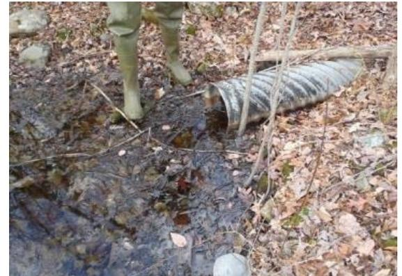
*This undersized culvert at the Maple St. crossing of the Segregansett River restricts water flow and fish passage.
