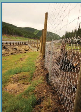
Photo 5: Installation of Reconyx cameras in the wildlife passages Photo 6: Large-fauna fence (top part) and medium-sized fauna fence (bottom part)
